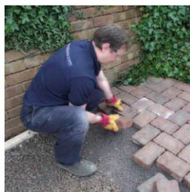
**STEP 3:** Bradstone Infilta blocks have a nominal joint width of 5mm which is greater than normal block paving
