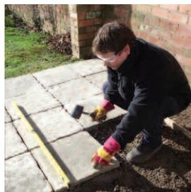
Trowel the mortar into the joints, pressing it down and smoothing over using the pointing bar if necessary.
